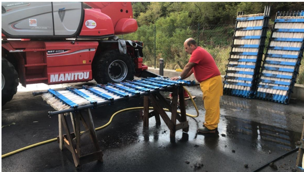
Fig.4 removal of air nozzles for one membrane row
