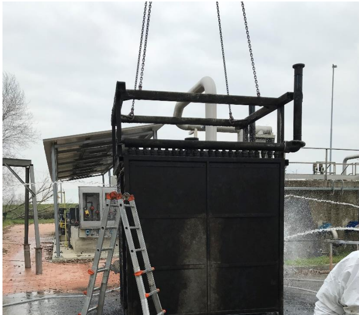
Fig.1 chains used to lift the module from the tank
